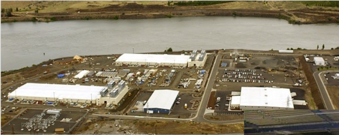
Google's Datacenter in Oregon
